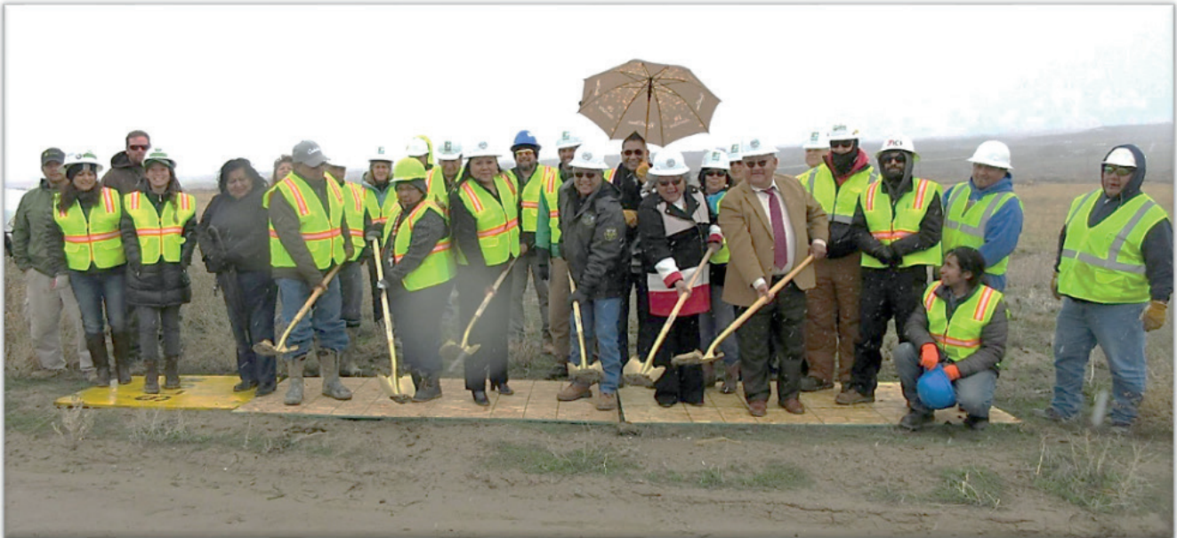
Figure 7. Ute Mountain Ute Tribe Officials and Grid Alternatives begin the construction phase of a $2 million solar array. Source: Cortez Journal, March 15, 2019
